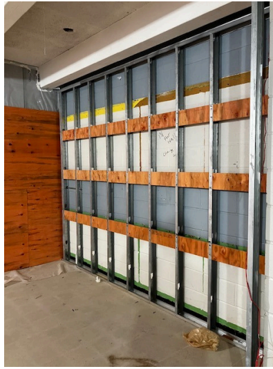
Wall blocking installed between the steel studs in one of the classrooms to support the new cabinets.
