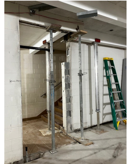
Temporary posts supporting the floor beams above the Music Room on the First Level.
