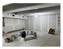
Drywall on the 2 nd Level of the 1961 Addition is nearly complete and crews are well along with taping and mudding the joints.
