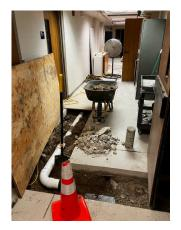
The new sewer pipe for the classroom sinks continues down to the Corridor outside the Fellowship Hall Kitchen where it ties into the existing sewer main.
