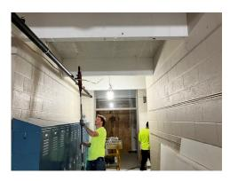
The suspension grid for the lay-in ceiling is starting to be installed in the 2nd Level Hallway of the 1961 Addition.
