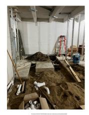
The concrete in the floor of the Music Room has been sawn, trenches dug and sewer pipe being installed for the sinks in the six classrooms in the 1961 Addition of the School.
