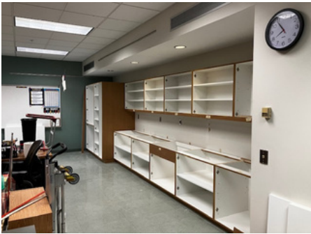
Olson Cabinets, who is making all of the cabinets for the project, has started installing cabinets on the second level of the 2000 addition. Since they were constructed 25 years ago, these classrooms never had cabinets or sinks.
