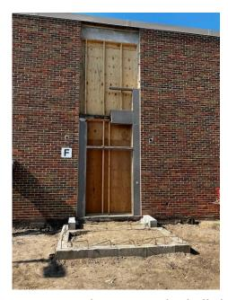
The concrete foundations were backfilled this week. The South Entrance door and window frame is being removed so that the new vestibule addition can be built.
