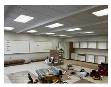
The interiors of the Second Level classrooms in the 1961 are nearing completion. The vinyl composition floor tile has been installed, walls painted, ceilings and the new lighting installed. Installation of the new cabinets is moving well along. Interior finishes in the First Level of the 1961 Addition are following about a week behind those in the Second Level.
