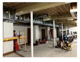
With much of the work being completed in the school portion of the project, work is picking up again in the Fellowship Hall. The main trunk ductwork has been installed and the soffits around them are being framed. Under slab plumbing for the new Fellowship Hall Toilets is also underway.
