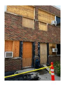
Framing and waterproofing for the new air intake louvers for the HVAC ventilators in the 1961 addition are being installed. The new louvers will be much larger than the previous louvers because the new units will be mixing in more outside air, so that the air in the classrooms will be much healthier than it was previously.
