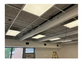
The floor trenches for the sewer lines for the new classroom sinks have been infilled with concrete. The new steel column and beams which support the floor above the new passageway north of the Music Room have been installed.
