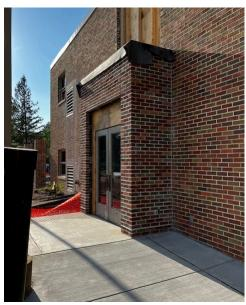
Brick has been installed on the South Entrance Vestibule projection. Until new doors are installed and the interior is finished, use these doors for emergency egress only.
