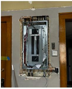
The old (possibly original) electrical panel in the Vestry has been removed and is being replaced. All panels, wiring, and devices in the renovated areas are being updated with new ones.
