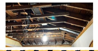
The original plaster and later tile ceilings in the Vestry and Sacristy have been removed to allow for insulation. New gypsum board ceilings will match the original vaulted design.
