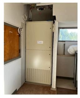
The classroom unit ventilators have arrived, and the first is being installed. These units provide heating, cooling, and ventilation to the six classrooms in the 1961 Addition, with energy recovery wheels to temper incoming fresh air using exhaust air.
