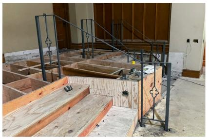
The steel portions of the new raised Chancel railings have been installed. Hardwood caps will be added to the tops. The space under the raised floor will be filled with insulation to reduce walking noise.
