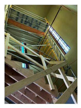
Now that the new balcony stair has been framed, scaffolding has been erected on top of it to access the church attic. The existing contaminated attic insulation will be removed and replaced with new insulation and fire sprinklers will be installed in the attic to protect the Sanctuary.
