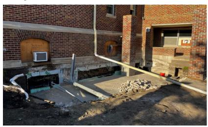
The area at the removed coal bin has been backfilled. Because the structural capacity of the original basement wall is unknown, the engineer required that the void be backfilled with lightweight lean concrete fill, so no lateral pressure is applied to the wall.
