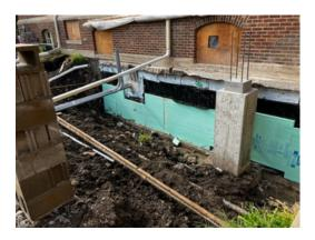
The opening in the basement wall where the coal bin was previously has been infilled with concrete, waterproofed and insulated. There is a drainage tile along the footing which will be connected to a new sump and pump. The gray pipes are electrical conduits for new electrical service to the exterior HVAC units and for the new electrical panels in the Boiler Room. The concrete column is for one of the posts for the screen wall around those HVAC units.
