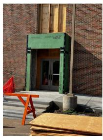
The small projection for the new south vestibule has been framed and sheathed; ready for brick. Due to limited space, about one third of the vestibule will be in this projection while the remaining two thirds will be inside the building. The vestibule will have wider doors which will allow access for individuals in wheelchairs.
