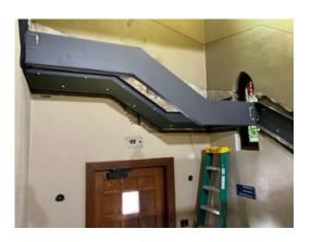
Iron workers are installing the structure for the new stairway up to the Balcony. The structure for the stair is steel, but all exposed portions of it will be white oak, in the style to match the original stair. The new stair will have safe treads instead of having dangerous winder treads, which the original stair had.
