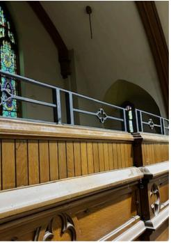
Installation of the balcony railing underwav. extension is extension is lower and as open as possible to allow better visibility. The metal portion of the extension will be painted a darker bronze tone and an oak cap will be added.
