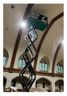
The fire sprinkler contractor has started cutting holes in the plaster ceiling for the sprinkler heads. These heads will be recessed and covered with flush caps.
