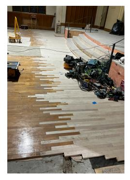
The wood flooring contractor has extending the maple finished flooring to the base of the Chancel. They have now begun removing the portions of the existing floor that were damaged by water leaks over the years.
