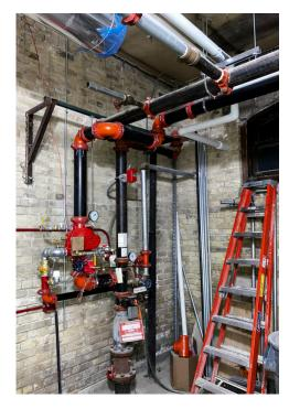
A dry system valve has been added to our existing fire riser in the basement storage room under the Sacristy. This valve keeps water out of the pipes in the attic and other cold areas, until a sprinkler head calls for water.
