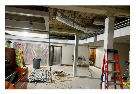
Sheetrock is being installed on the soffits in the Fellowship Hall, as all of the above-ceiling work in those areas is complete.
