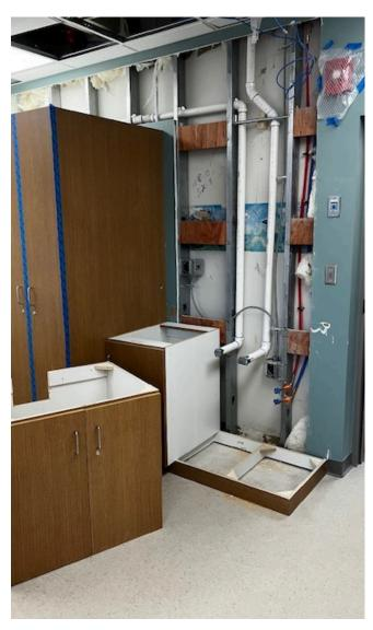
Over Christmas break, the sink is being installed in the Nursery/Preschool Room. This sink will have a lift to remove the waste, because the floor could not have been cut, due to existing electrical conduits in the floor.
