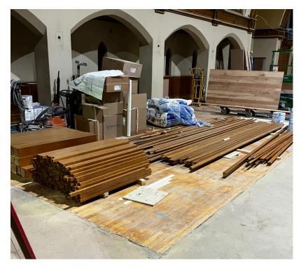
Some of the oak trim for the Sanctuary arrived this week. Most of it is prefinished. The panels going into the side aisle wainscoting is not. It will be stained in place to match the existing adjacent panels.
