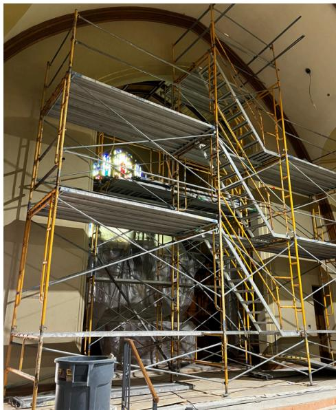
Scaffolding has been set up on the raised Chancel floor to repair and paint the plaster ceiling and varnish the woodwork. In the remainder of the Sanctuary, that work will be done from a lift instead of from scaffolding.
